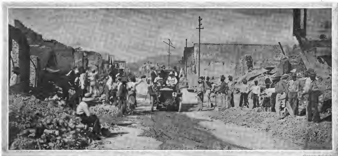
EAST STREET, ONE OF KINGSTON'S THOROUGHFARES AS IT LOOKED AFTER THE EARTHQUAKE HAD DONE ITS DESTRUCTIVE WORK.
